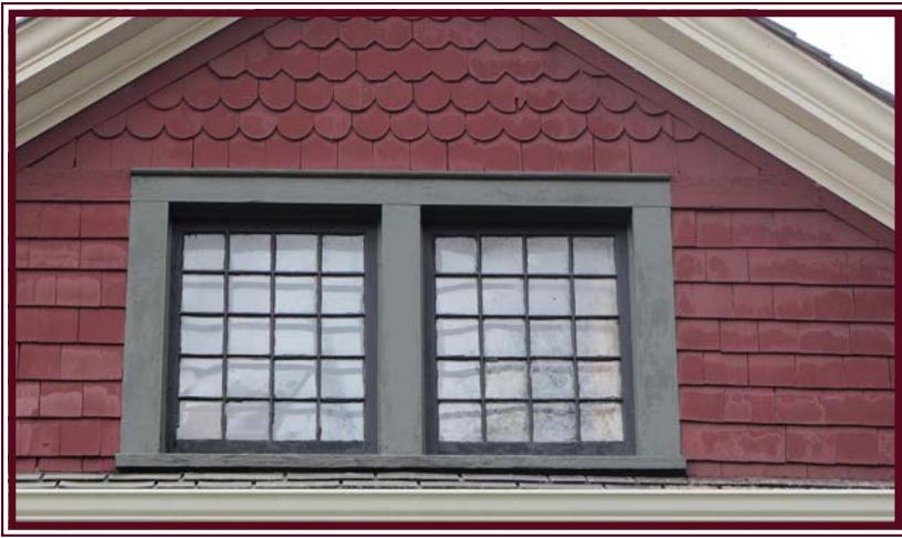
View of attic windows, west facade. Source: Artifacts Consulting, Inc.
