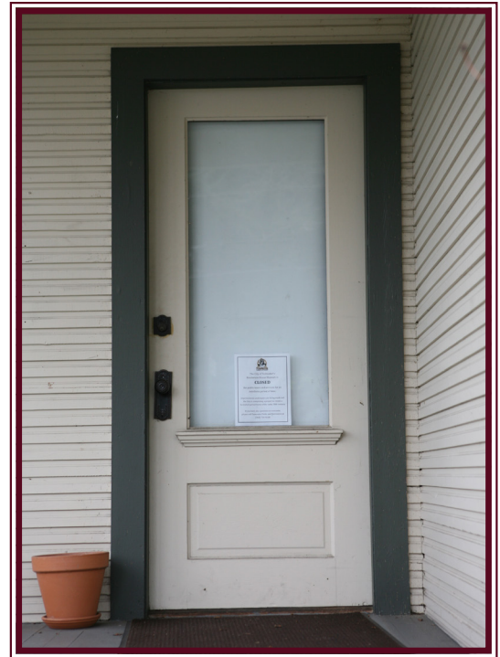
View of front door, located on west facade. Source: Artifacts Consulting, Inc.
