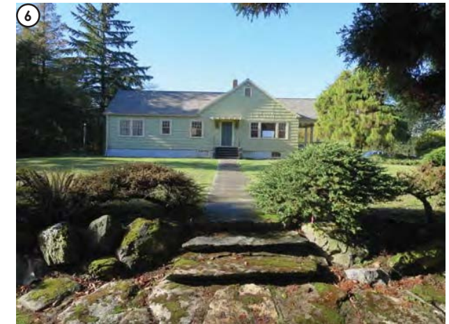
6 Stone slabs still serve as steps, concrete walk beyond. No plantings at house remain. (11/16, KKLA)
